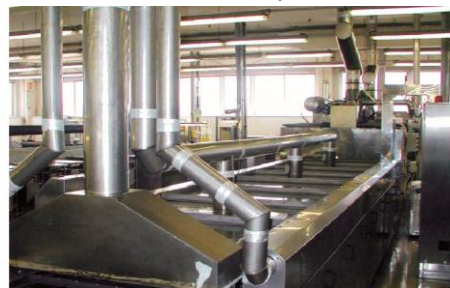
Industrial vessels and storage tanks
